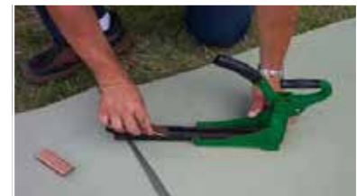
Loading staples into the manual staple gun
