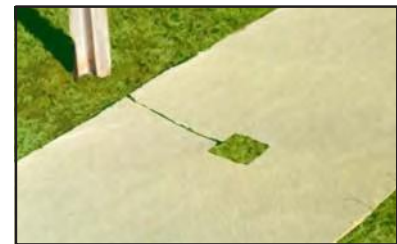
If there is an existing guardrail in place, slit the material from the hole to the edge
