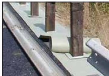
Cutting the WeedEnder™ roll when the pre-punched holes do not match post spacing.
