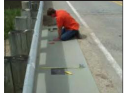
Installing WeedEnd™ to existing guardrail
