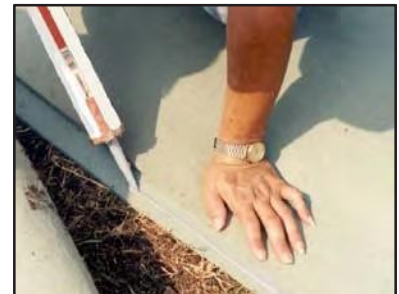
Applying Adhesive Caulk to the Joining Strip
