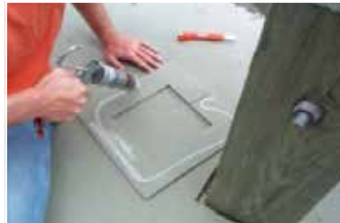
Applying caulk to the footprint
