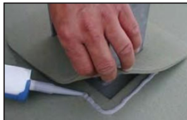
Applying a bead of adhesive caulk to the footprint
