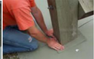
Pressing the footprint firmly into position
