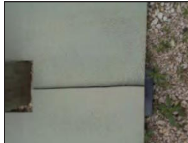
After opening the slit at each guardrail post slide the WeedEnd™ around the post
