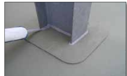
Applying a bead of adhesive caulk around the guardrail post
