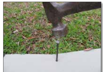
Stake the material in place
