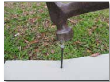
Installing the spikes along the edge of the WeedEndeR™ material
