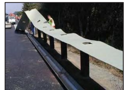
Prepunched WeedEnder™ roll being placed over guardrail posts
