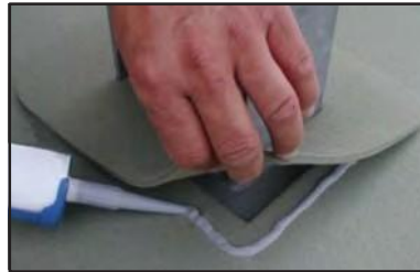
Running a bead of adhesive caulk under the footprint
