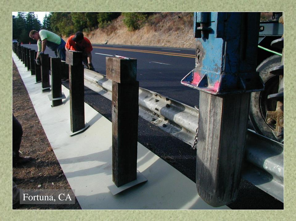
The installation of the WeedEnder® system is completed by installing post collars to eliminate the growth of vegetation around the guardrail posts. Collars for all post sizes and profiles are available and are provided for each project.
