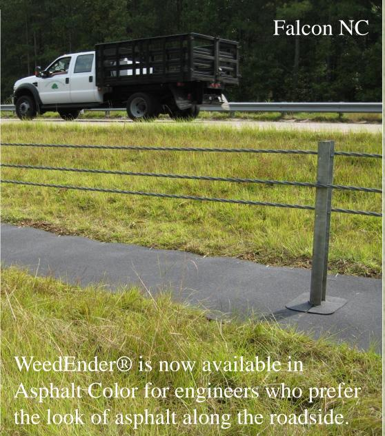
WeedEnder® is a very safe option for guardrail or cable barrier treatments where new plantings are present as well as near sensitive agricultural zones where over-spraying or drift from herbicides can be risky.
